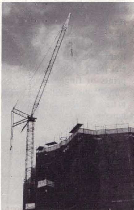
A Manitowoc 3900 mobile tower crane on hire from Brambles Cranes to Concrete Constructions for use on their Bondi building project.
